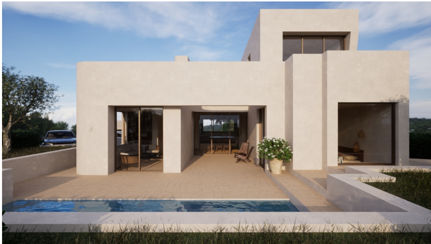
South façade - Pool terrace
