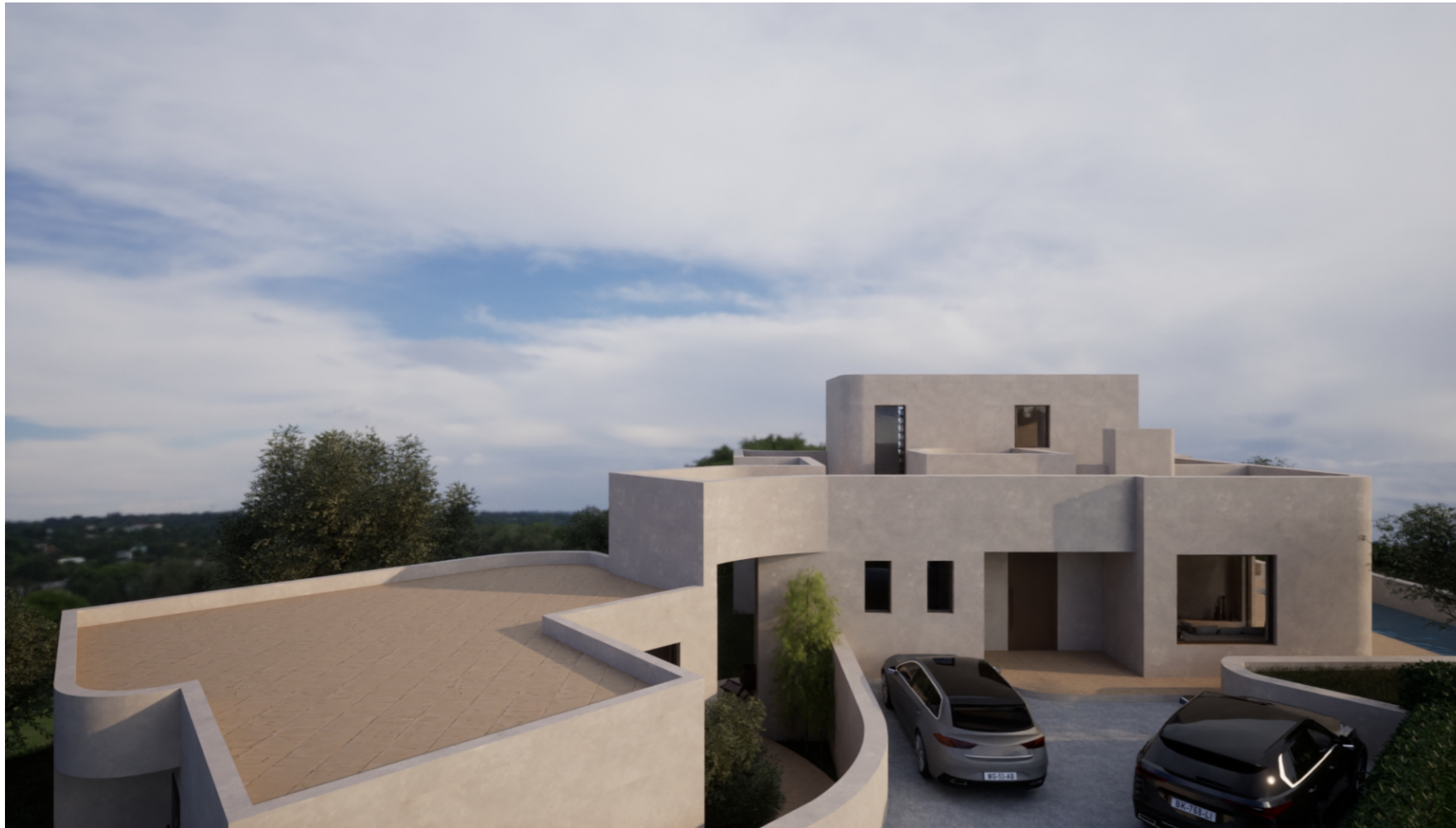
General west view of the flat roof terraces.
